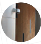
Exterior panel joints
